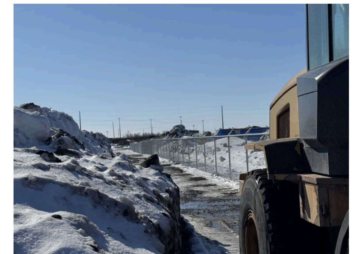
Station Site Prep at Yates Ave. (grubbing, soil preloading, fencing installation)
