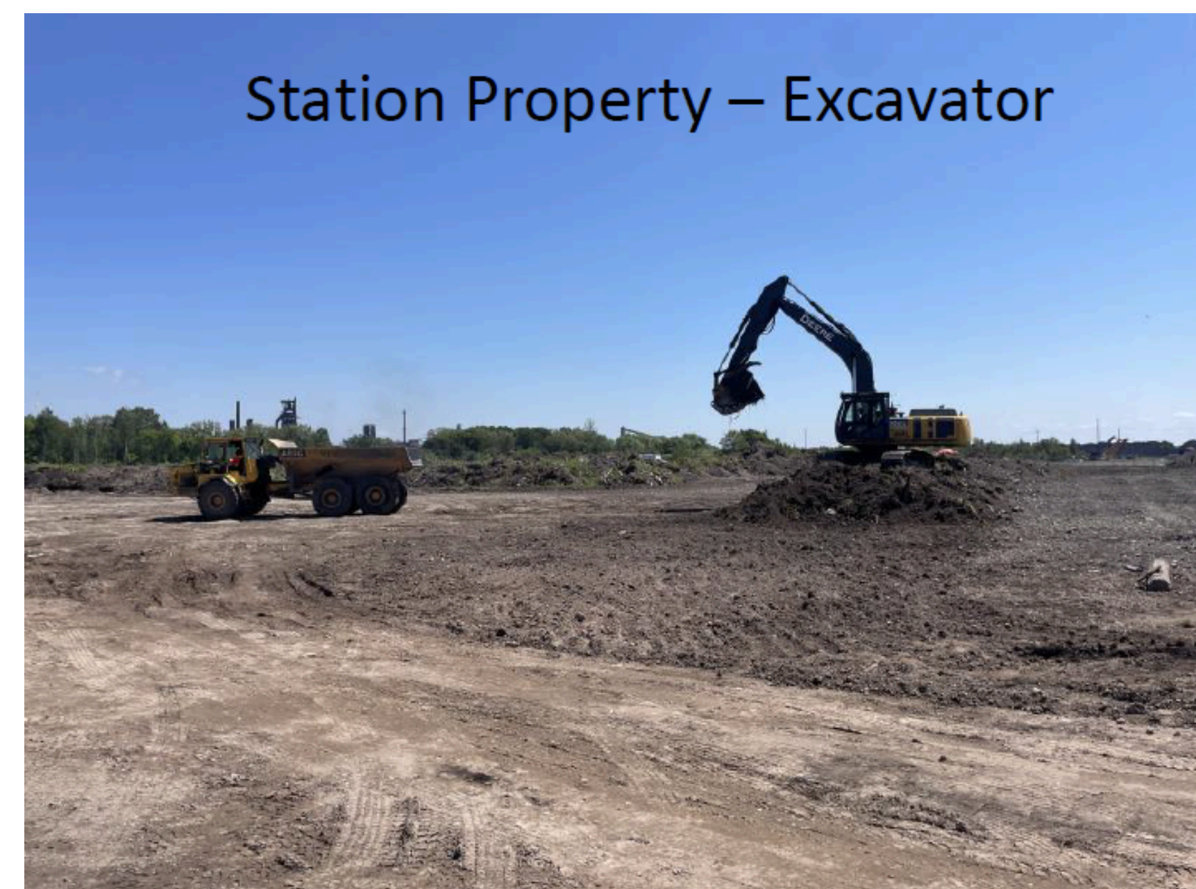
Station Site Prep at Yates Ave. (grubbing, soil preloading, fencing installation)
