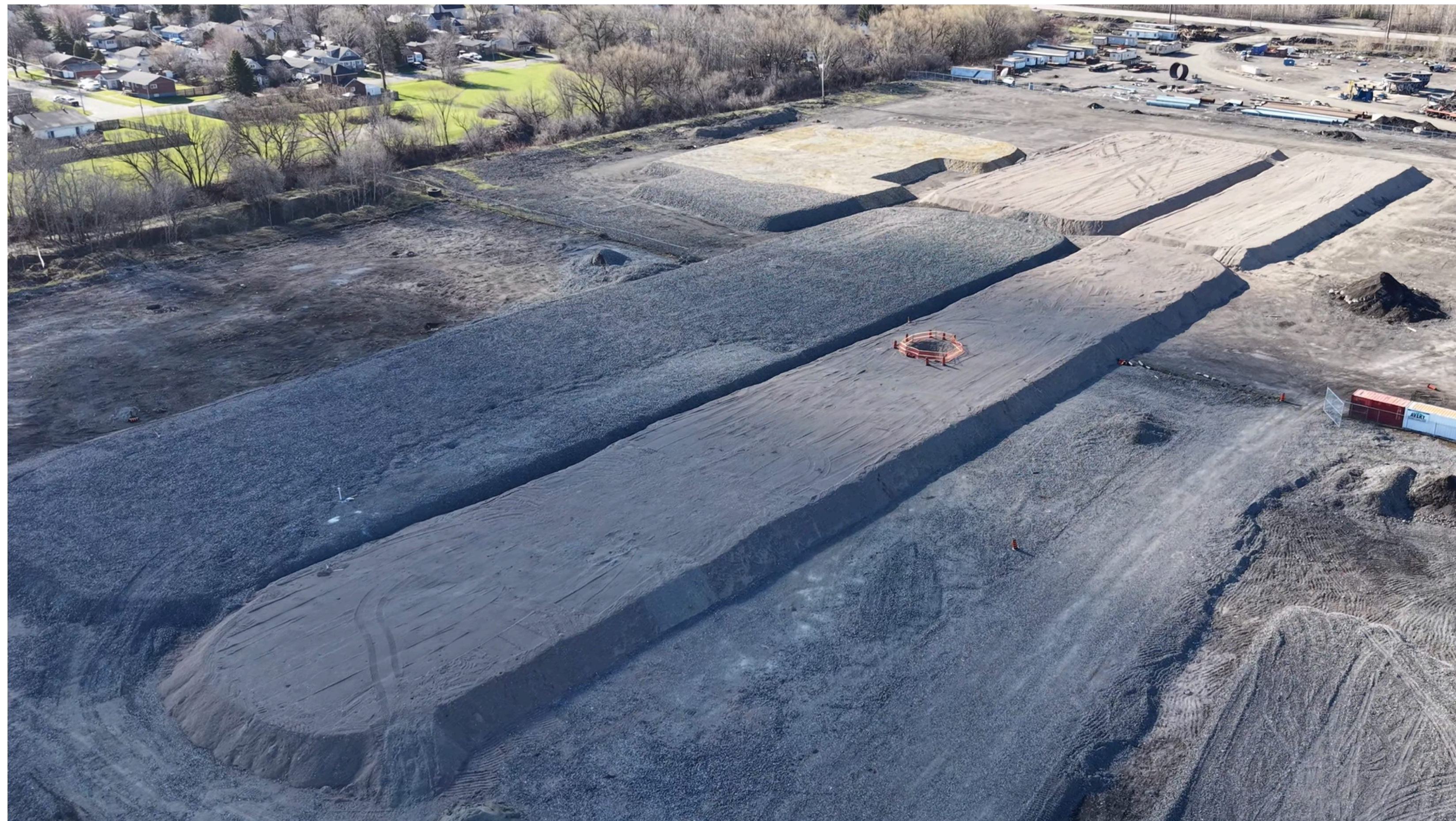
Station Site Prep at Yates Ave. (grubbing, soil preloading, fencing installation)
